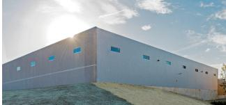
An addition to an existing ABC building, this expansion includes a 29,000 sf manufacturing area with an office. The office features a full mezzanine with an attached 1,112 sf Ecospan deck. The exterior is constructed with a combination of precast panels and the HE40 Heavy Embossed insulated metal wall system, and a 27'6" surrounding parapet.
