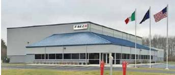
rib standing seam. The office buildings feature horizontal ST40 Striated insulated metal panels, masonry wainscot, ribbon windows, and skewed corner.
