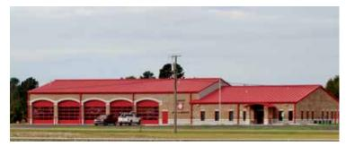
two buildings without endwall columns blocking numerous walk doors between the two sections.
