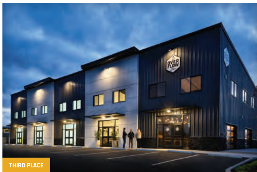
② PowerCo, Inc. Bethlehem, PA BUILDER: Schlosser Steel Buildings, Inc.
