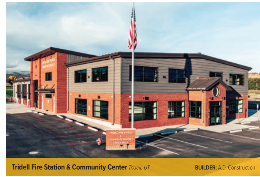
Tridell Fire Station & Community Center Tridell, UT
